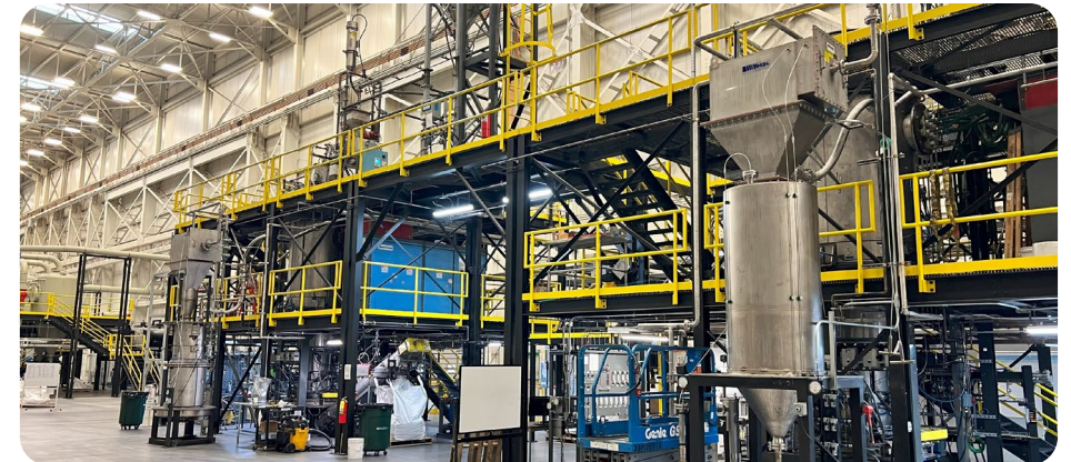
NOVONIX Riverside Facility in Chattanooga, Tennessee Facility to scale to 20K tpa aligned with customer demand
