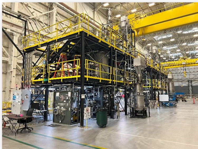
Figure 1 NOVONIX Riverside Facility, Chattanooga, Tennessee
