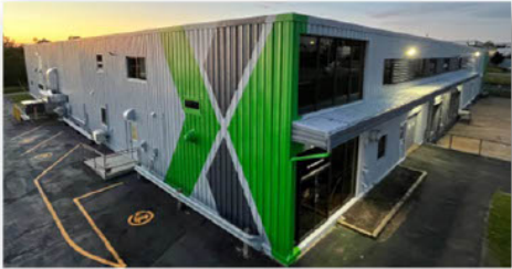
NOVONIX Simmonds Facility in Nova Scotia, Canada
