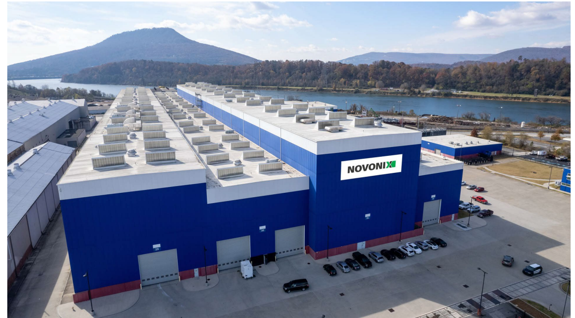
Riverside Facility in Tennessee
