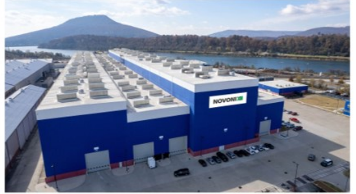
Riverside Facility in Tennessee
