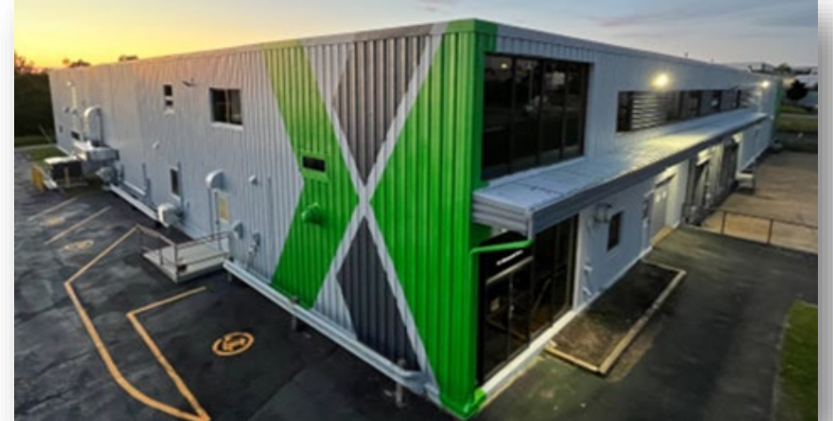
NOVONIX Simmonds Facility in Nova Scotia, Canada
