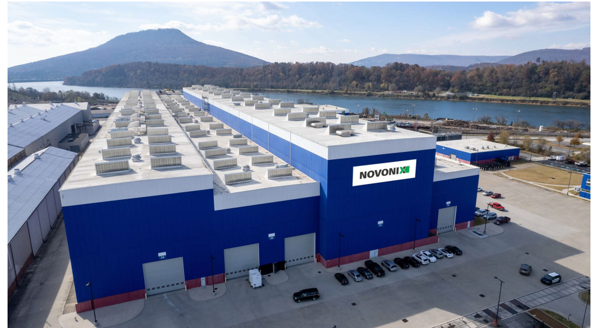
Riverside Facility in Tennessee
