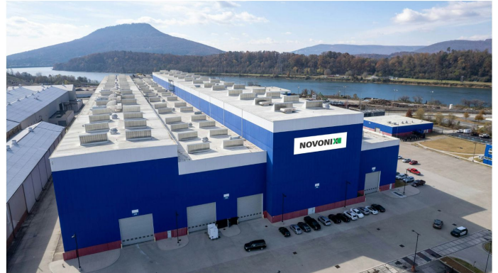
Riverside Facility in Tennessee
